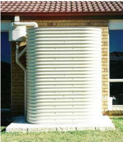
The picture adjacent shows a typical rainwater tank only collecting part of a roof. The downpipe connects directly to the top of the tank. This is the most ideal installation. However, due to the Basix Tool penalizing collection of only part of a roof, most clients choose the entire roof area to drain to the tanks, other wise the tank size is increased in size to volumes that must be put underground.
