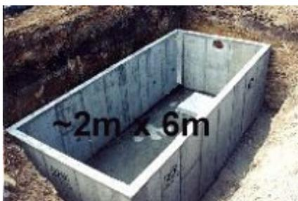
The picture to the left is an underground tank, before the concrete lid and access grates are constructed. Their depths vary, based on your site conditions.
